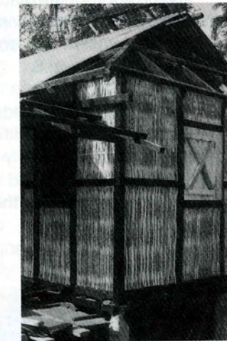
Fig 3 House built of especial type of reeds, eventually to be plastered with mud or cement, extensively used in Sylhet region, Popularly known as Ekra wall, is hardly known to students even professionals.
