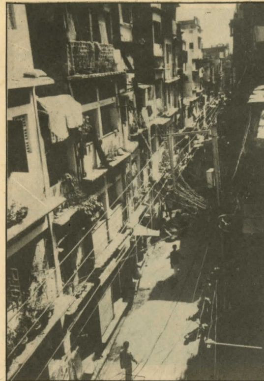
Narrow Street of Shakharee Patti Defined by Building Line
