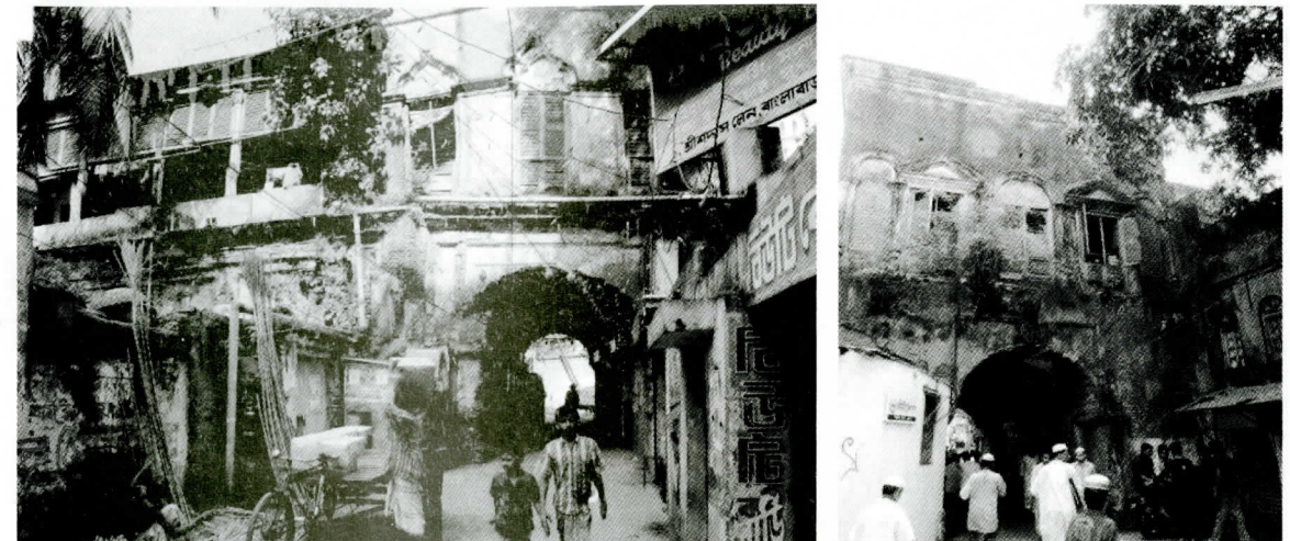
Fig 20: 1, 2_Shirish Das Lane_ arched approach acts as a gateway.
