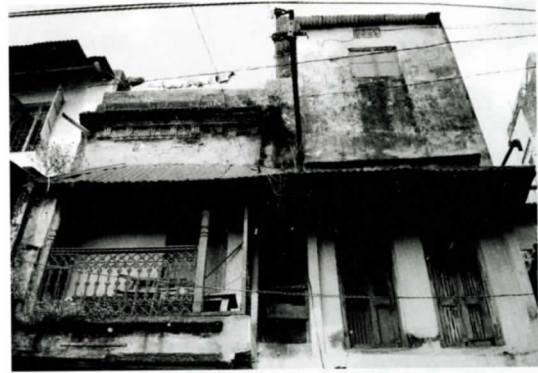
Fig 10: Extension work is common feature
