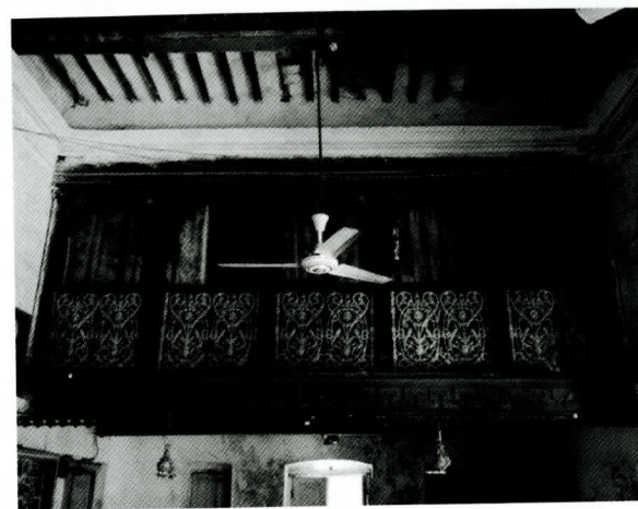
Fig 30: Wooden lattice work in the balcony
