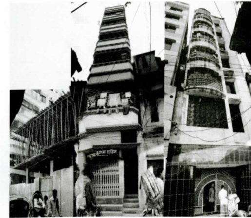
Figure 04: Old structures are being replaced with new 6 storey buildings
