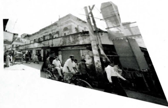
Fig11: Use is replaced - residence-turned into storage space
