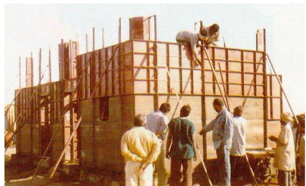
Figure 18: Rectangular house under construction in 2001 Kutch earthquake rehabilitation exercise. Source: Kotak, 2007, p70.
