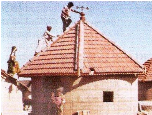
Figure 17: Circular house under construction in 2001 Kutch earthquake rehabilitation exercise. Source: Kotak, 2007, p71.
