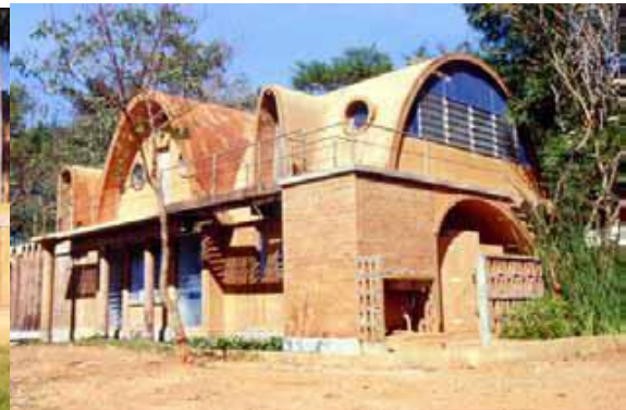
Figure 20: Training Centre at the Auroville Earth Institute, Various vaults with stabilized earth waterproofing Source: Maini, 2005.
