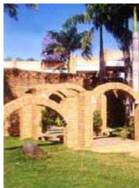
Figure 19: Arches of the Visitor's Centre at Auroville, CSEB Technology. 1992 Hassan Fathy Award for Architecture for the Poor. Source: Maini, 2005.
