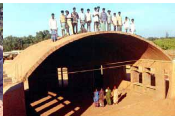
Figure 22: Vault of Mirramukhi School at Auroville, CSEB. 10.35m span, 2.25m rise, 30 tons – Built in 3 weeks Source: Maini, 2005.
