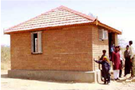
Figure 15: Houses built by the CRS – Gujarat, India. 2698 houses built in a year time, in 39 villages. Source: Maini, 2005.
