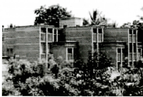
Figure 23: Staff quarter of the Health Centre. CSEB Technology. Source: Maini, 2005.
