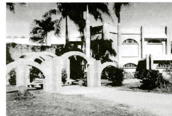
Figure 19: Arches of the Visitor's Centre at Auroville, CSEB Technology. 1992 Hassan Fathy Award for Architecture for the Poor. Source: Maini, 2005.
