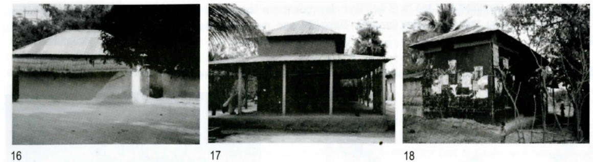
Fig. 16: Large overhang is used to protect the mud wall.
