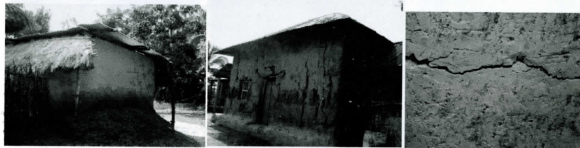
Fig. 13: The moisture rising from the ground make the earthen wall wet.
