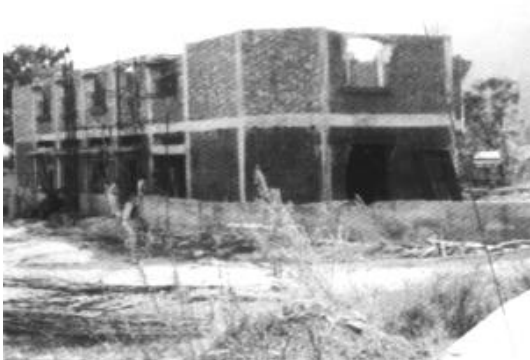
Figure 06: Earthquake effect on Frame and Non-frame structure
