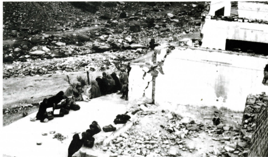
Figure 03: Destruction of a School in Bagh Town during the Earthquake in 2005
