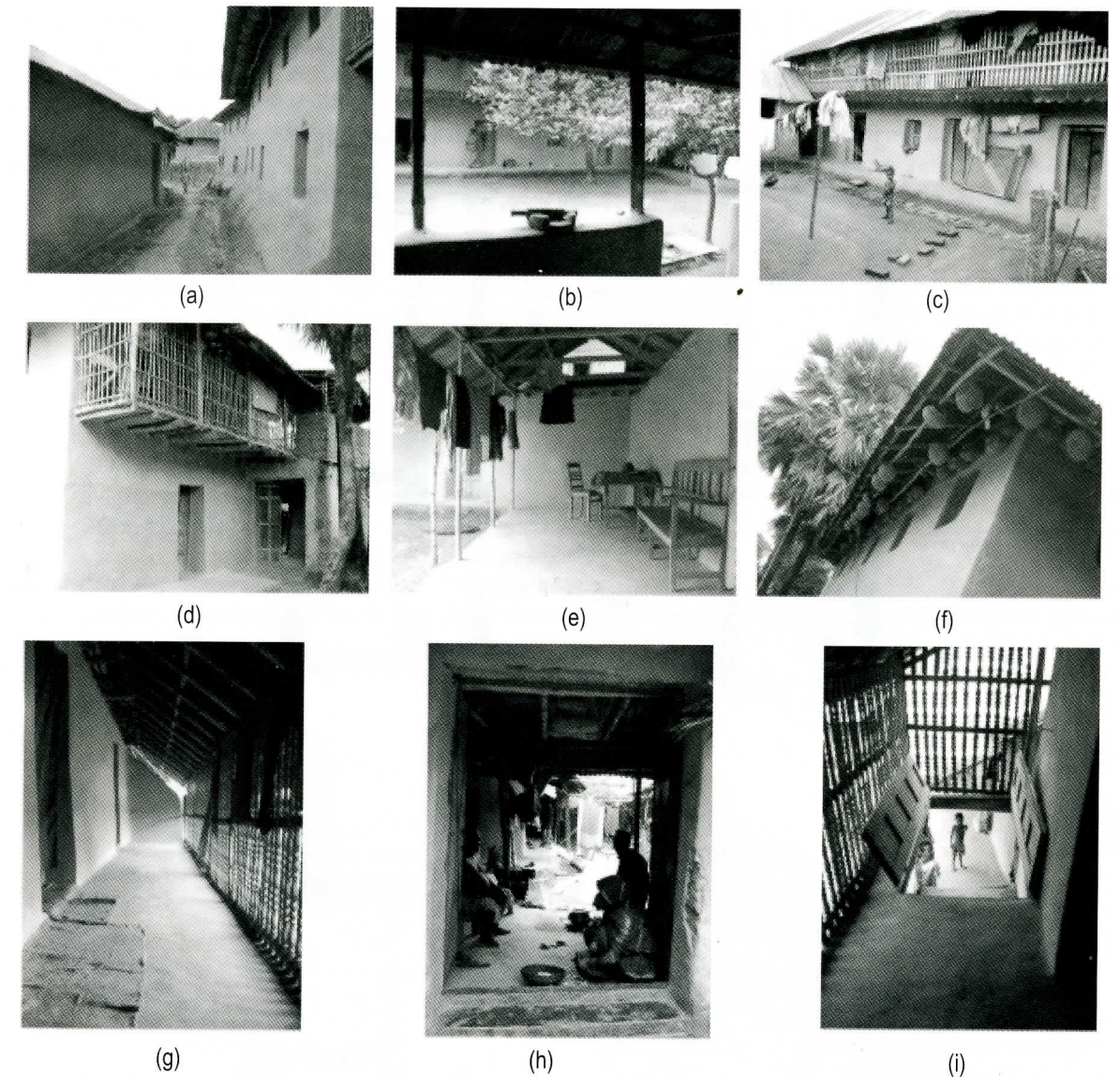
Figure: 02: (a) DO-MAHELA & neighborhood, (b) view to courtyard, (c) court facing two-storied façade and cantilever PIRA SAJANNI, (d) cantilever balcony and other details, (e) AKSAALI and spatial relation, (f) hanging bird nest, (g) hanging veranda, (h) space beside kitchen & (i) JAHAJI DHAP or single-flight wooden stair
