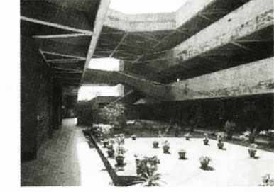
Figure 15: Bangladesh Agricultural University, Faculty of fisheries. The open-air courtyard in between the lecture theatres – an effort by the architect to relate the courtyard, the study area and to solve climatic problem. Source: Author's photograph, 2002.
