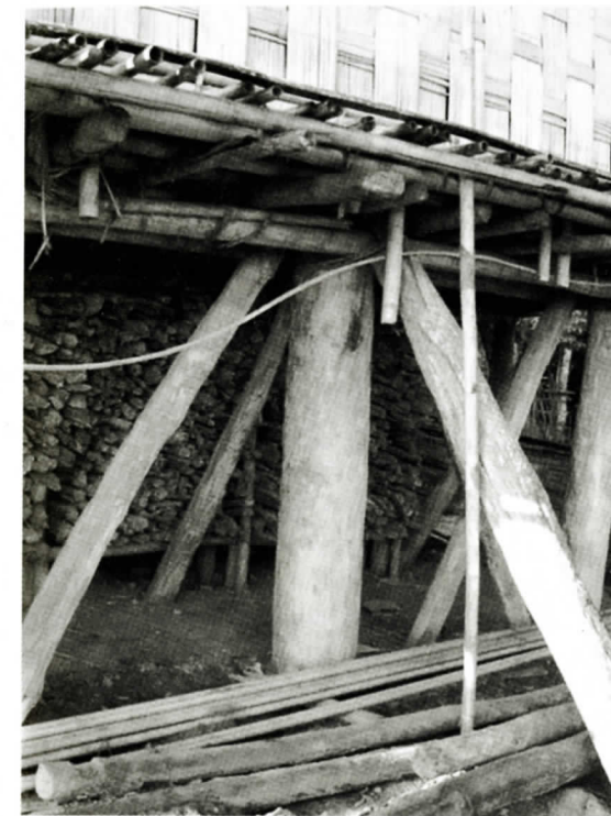
Figure 6: Stilt construction in wood. Hardwood trees with barks removed are used as posts. Bandarban 2003; photo: authors.
