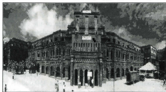
Figure 2 : The Chittagong Court Building
