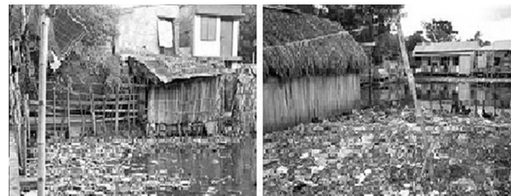
Figure 10: Adjacent water body is used as household waste dumping zone (Source: MSCHS Studio 2016-17).
