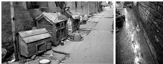
Figure 08: a) Covered drain and (b) open-drain used as wastewater discharge of the Rupsha slum (Source: MSCHS Studio 2016-17).
